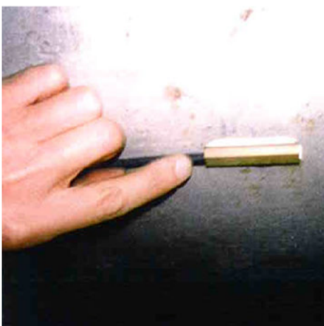
Figure 3 – Surface Temperature sensor installation on pipe
