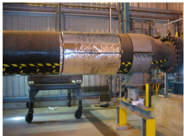
Figure 4 – Temporary insulation of temperature sensors
